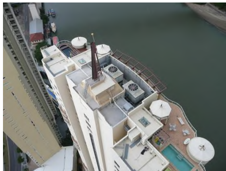
Figure 9. View from penthouse balcony to adjacent high rise tower roof
