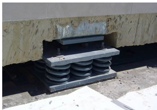
Figure 6. Swimming pool isolation system
